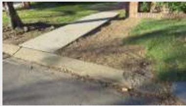
Local residents raised a request to rectify a path in Haslewood Court. The path was poorly sloped making it difficult for the elderly, bike riders and prams to negotiate. This resulted in many users “cutting the corner” eroding the surrounding area and increasing soil runoff into the lake. GCCC responded to the request with an improved design.
